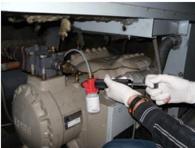
If there is no sampling valve on the tank, a tube and suction pump are used. The tube can be inserted into the vent opening each time (but this can be awkward) and likely contaminate the oil sample as the tube brushes against objects both inside and outside the housing. It is far better to install the tube permanently. Sampling then becomes quick and easy, as one simply connects the pump to the end of the
